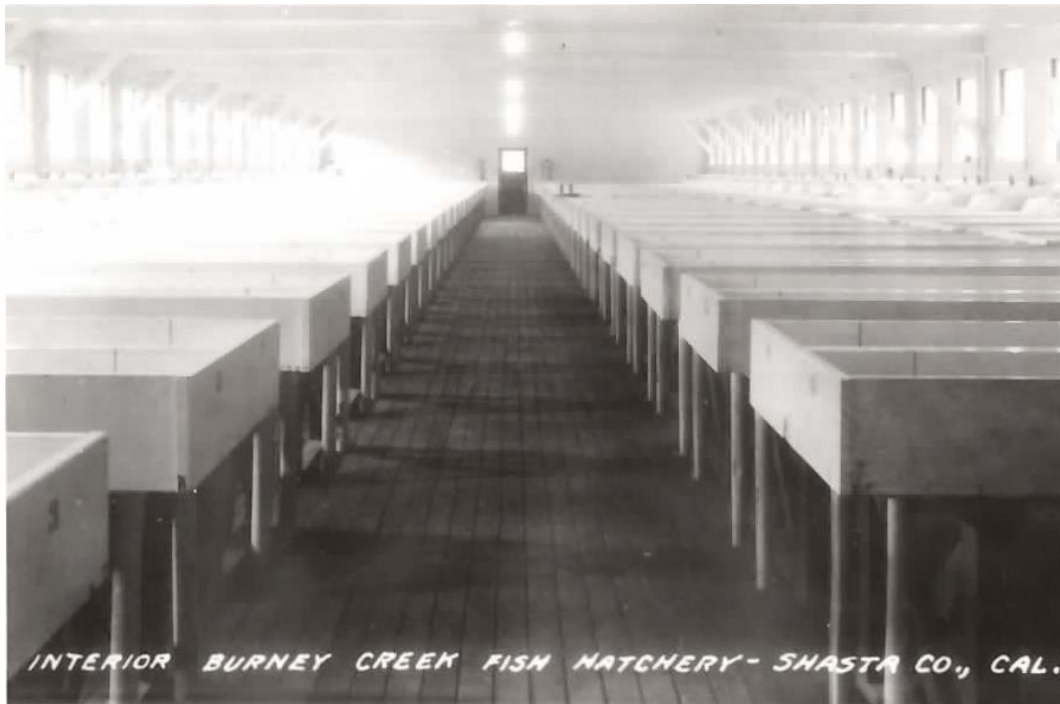
Interior Burney Creek Fish Hatchery, Shasta County, CA
