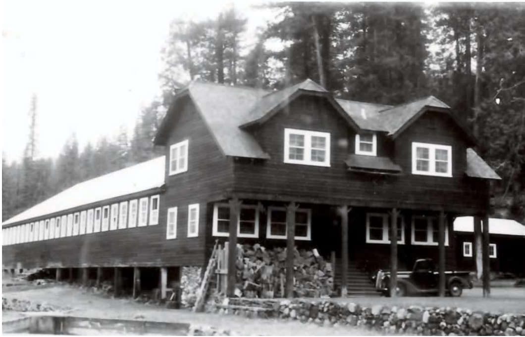
Burney Creek Fish Hatchery, Shasta County, CA
